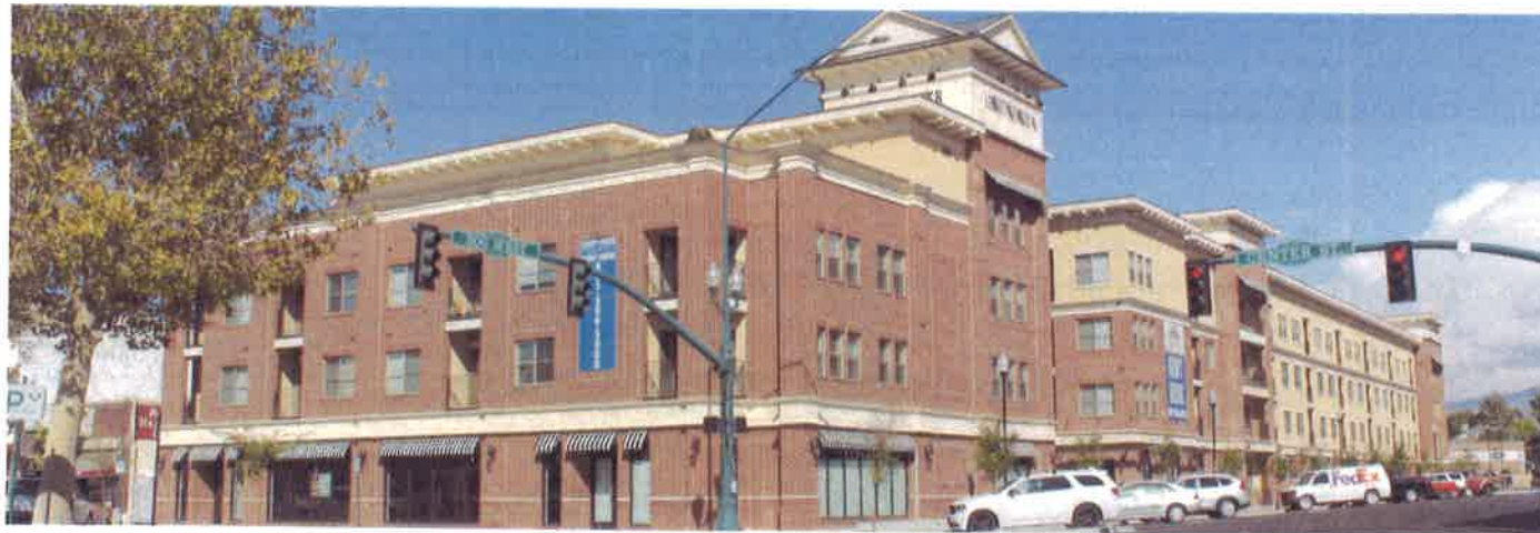
Liberty Center completed on 300 West between Center and 100 North
