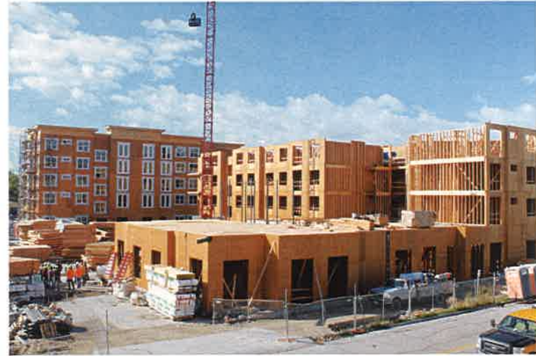
Pictured above, the Temple View Apartments under construction.
