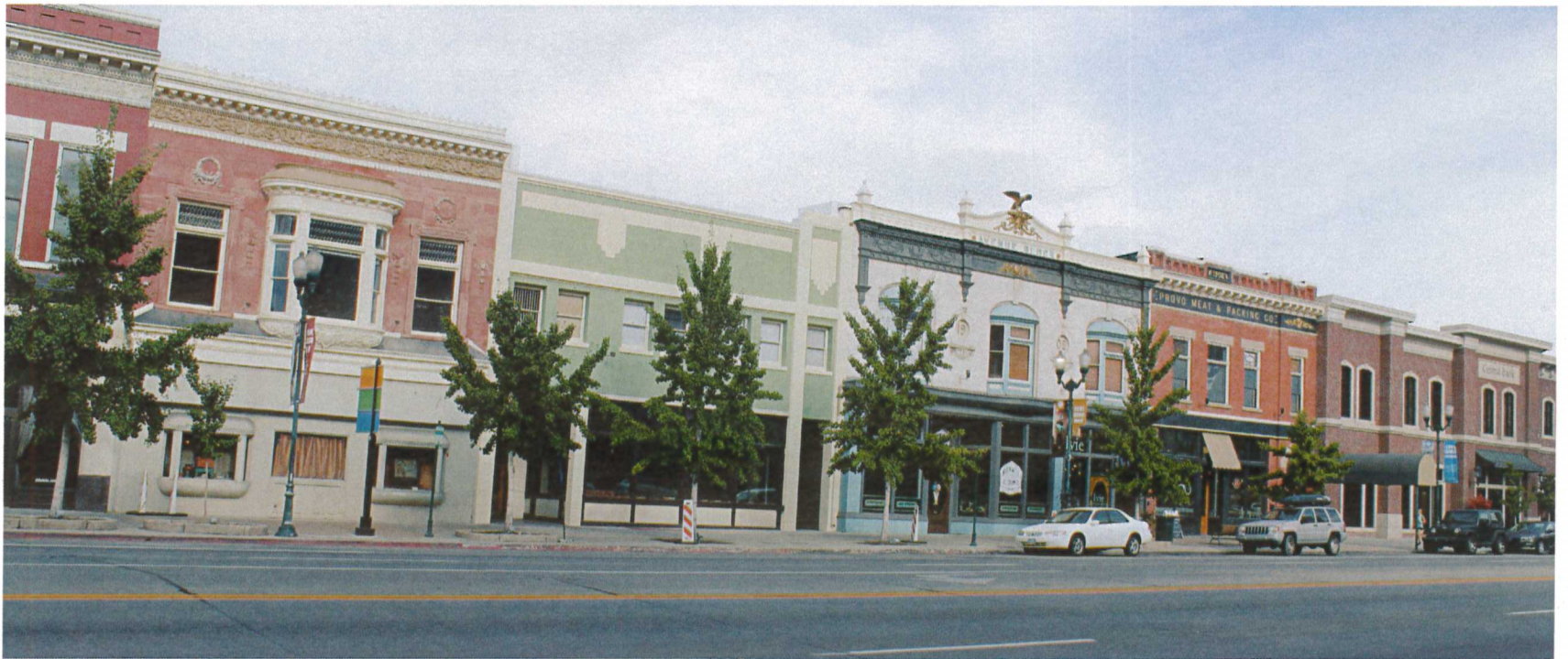
Pictured below, Provo Town Square buildings after façade renovation.
