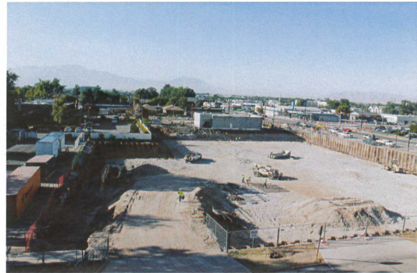
Pictured above, the site of the Temple View Apartments.
