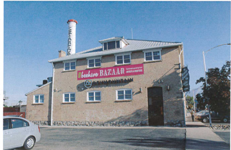
Start-Up building located at 600 South.
