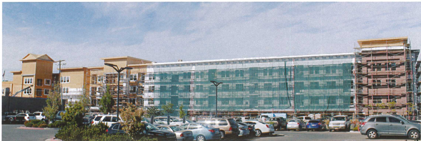
Liberty Center under construction on 300 West between Center and 100 North.
